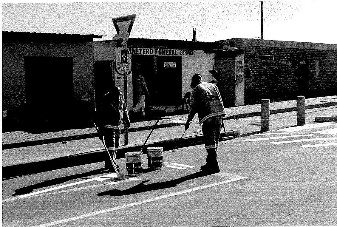
Image 8: Road marking in progress
