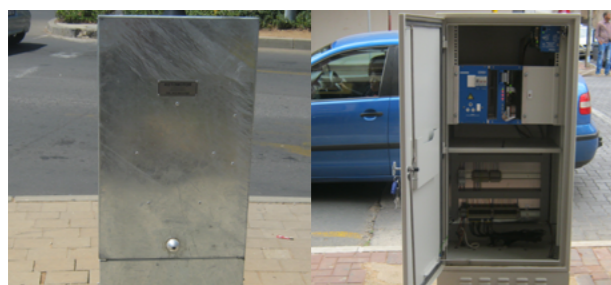
Newly erected automated controllers and Siemens controller boxes
