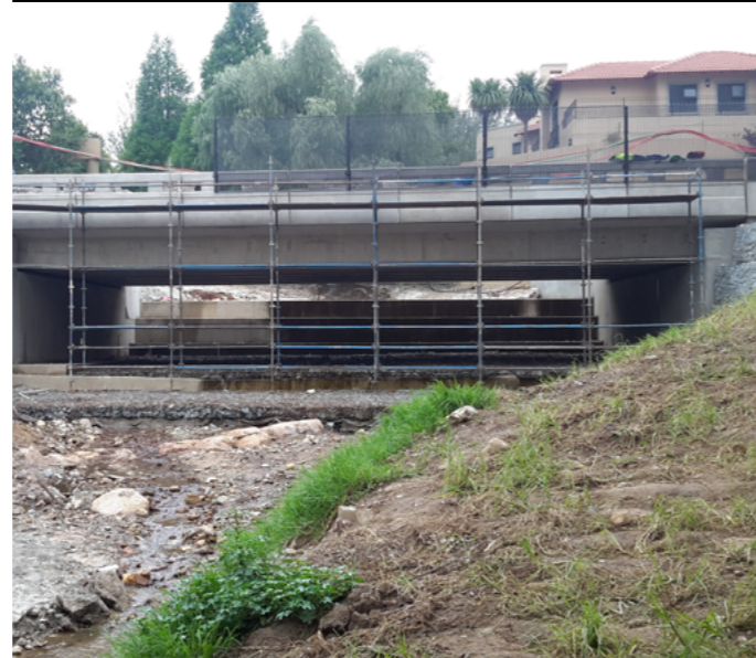
Near completion - Cornelius Road over Klein Jukskei River in Weltevredenpark
