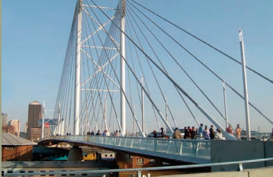
The Nelson Mandela Bridge
